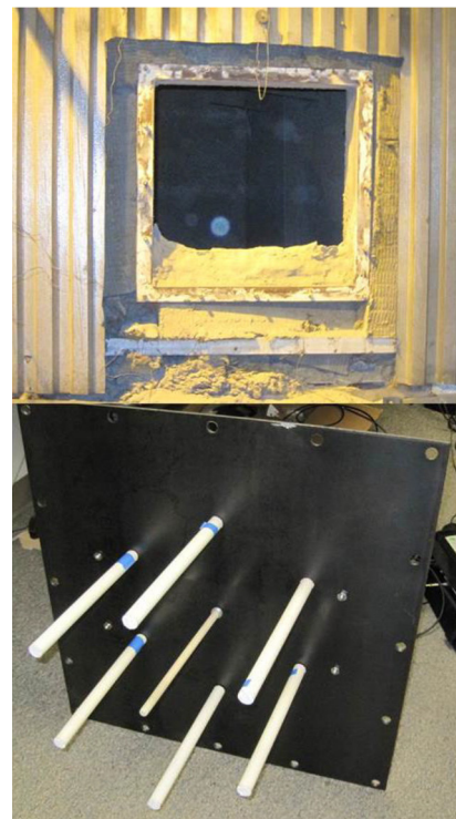
Access door to economizer area of trash burning boiler with array of six SAW sensors surrounding interrogation antenna in center.
